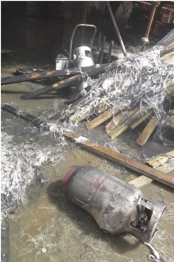
Fire initially involved scaffold containment mesh, formed of high-density polyurethane and fibreglass reinforced banding. The burning mesh separated and fell igniting fresh fires on lower levels and at ground level, adjacent to the basement. Fire intensity of the burning mesh was severe, resulting in fire entry into the basement and explosion of multiple stored gas cylinders within the basement.
