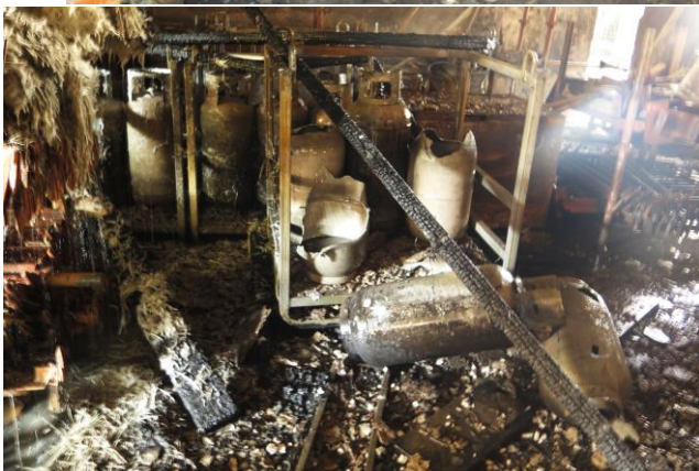
Fire entered the basement where gas cylinders were stored. Top left: LPG cylinders. Top right: Oxygen cylinders. Middle left Oxygen cylinders and projected LPG cylinders. Middle right: Oxygen and LPG cylinders used for cutting. Lower left: Breached LPG cylinders. Lower right: Stored diesel fuel.
