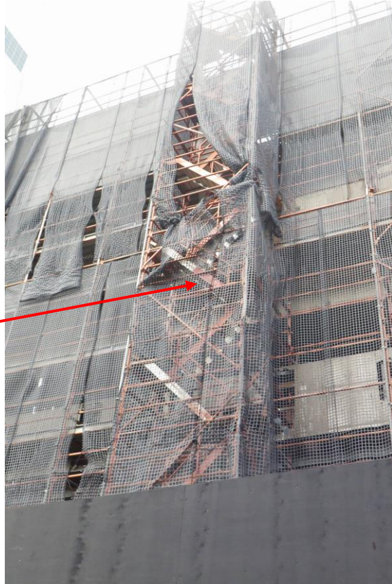
Upper: Ladder Platform 1 protected the structural steel that formed tower of the tower crane. Lower: Scaffold stairs located on the side of the building that enabled the workers to escape (indicated by arrows).
