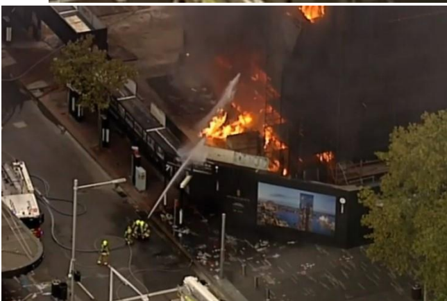
Gas cylinder explosions (Boiling Liquid Expanding Vapour Explosions/BLEVEs) occurred inside the basement. Several gas cylinders became flaming projectiles, travelling beyond the basement. These fire events are extremely dangerous. Firefighters used shielding and continued to fight the fire.
