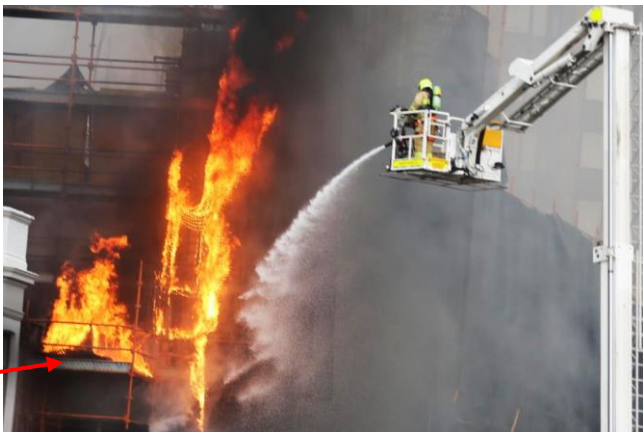
Ladder Platform 4 attacks fire burning within the Alpha side Scaffold mesh. Burning mesh has fallen and ignited combustible materials on the lower scaffolding A resulting in fire spread. The aerial streams achieved numerous incident objectives, including achieving fire containment, reducing fire intensity, extinguishment of spot fires and cooling of steel being impacted by fire (particularly the tower crane structure).
