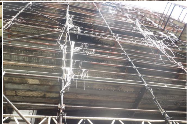
Fire initially involved scaffolding containment mesh, formed of high-density polyurethane and fiberglass reinforced banding. The burning mesh separated and fell igniting fresh fires on lower levels and at ground level, adjacent to the basement. Fire intensity of the burning mesh was severe, resulting in fire entry into the basement and explosion of multiple stored gas cylinders within the basement.
