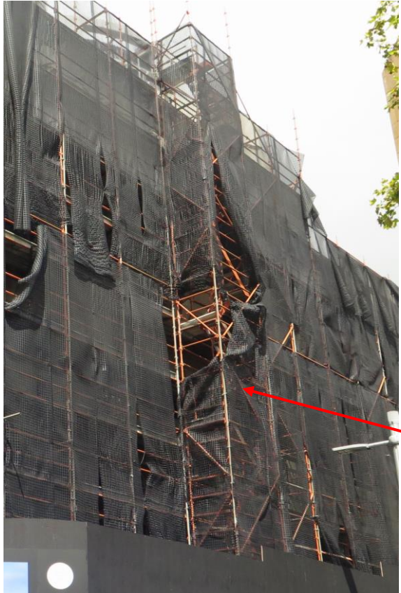
Upper: Ladder Platform 1 protected the structural steel that formed tower of the tower crane. Lower: Scaffold stairs located on the side of the building that enabled the workers to escape (indicated by arrows).
