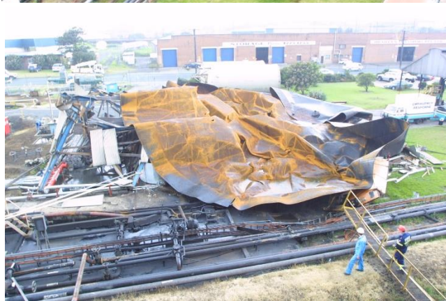
The 120-tonne fixed steel roof was blown off the storage tank by the force of the explosion and landed on the foam fire suppression system, rendering the system inoperable.
