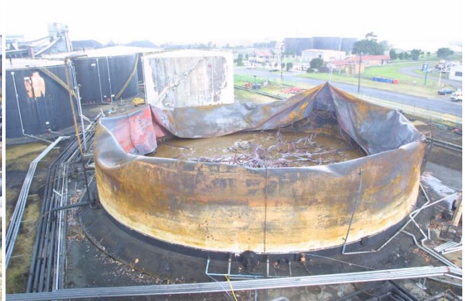
Upper: Twin headed attack hydrants were fitted to the site 150 mm diameter ring main. Radiant heat made operation of the ring main impractical. Middle: The burning ethanol tank was located in proximity to several storage tanks that came under significant threat. Lower (left) Attack hydrants were located on the bund wall. (right) The ethanol storage tank following extinguishment.
