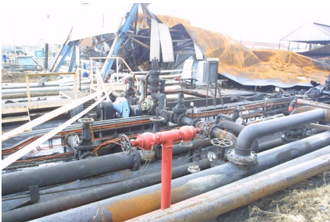
Upper: Twin headed attack hydrants were fitted to the site 150 mm diameter ring main. Radiant heat made operation of the ring main impractical. Middle: The burning ethanol tank was located in proximity to several storage tanks that came under significant threat. Lower (left) Attack hydrants were located on the bund wall. (right) The ethanol storage tank following extinguishment.
