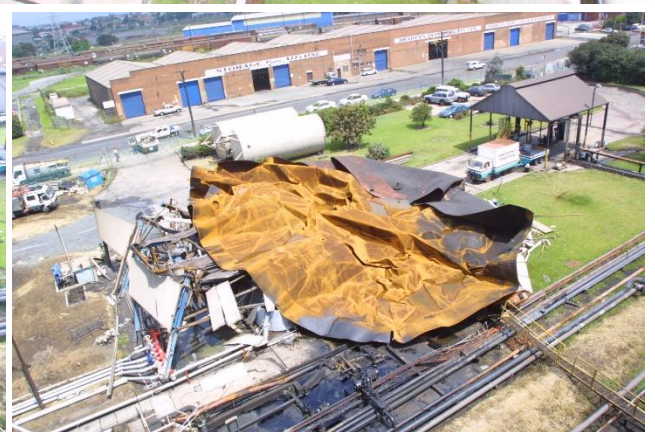
The 120-tonne fixed steel roof was blown off the storage tank by the force of the explosion and landed on the foam fire suppression system, rendering the system inoperable.
