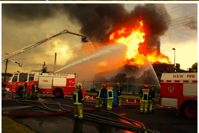
Foam Operations in Division A - Pumpers 52 and 54 supply foam to ground monitors positioned at the front of the storage tank. Firefighters were using ATC (Alcohol Type Concentrate) foam.
