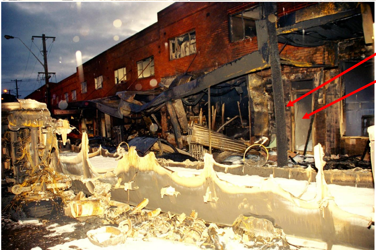
The entrance doors to units above the shops were completely impassable due to the fire, indicated by arrows. Heavy firefighting streams by initial arriving crews increased the survivability of the apartments above the entrance doors.
